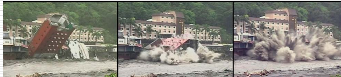
Collapse of a 6-story hotel in Taitung
